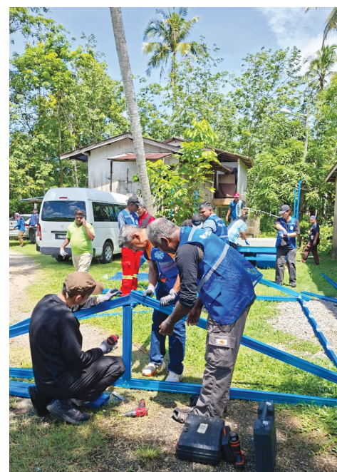
The volunteers working together to build 20 emergency flood rafts in Kelantan.
