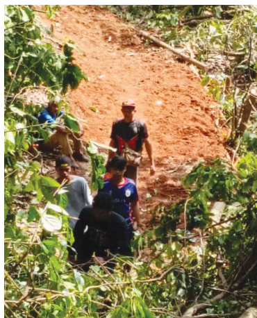
Volunteers clearing the land to lay the pipes.
